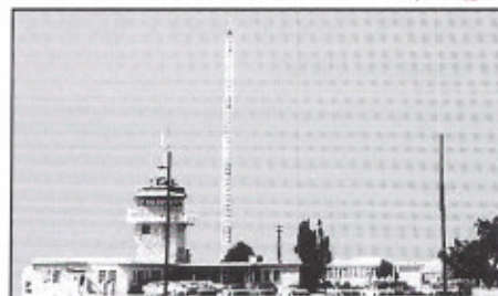
Aircraft tower that housed the W6FCS station
